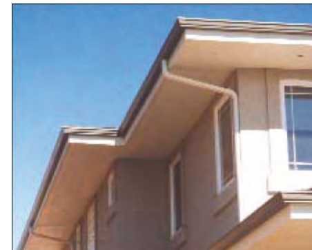
Deep overhang with flat soffit
