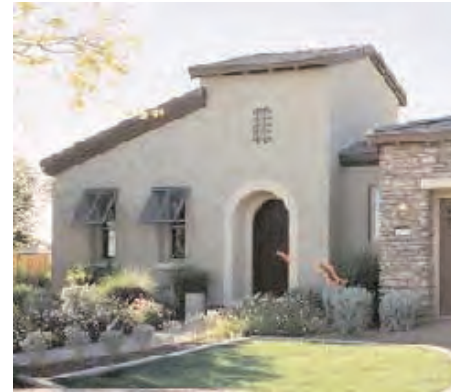
Typical Northern New Mexico house
