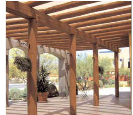
Rough-sawn wood details
