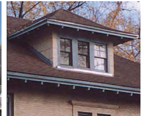
Hipped roof dormer
